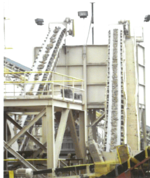
Conveyors from the primary (L) and secondary (R) crushers move material into hoppers that feed Telsmith 66 gyrasphere and Telsmith 57 SBS crushers, respectively.
